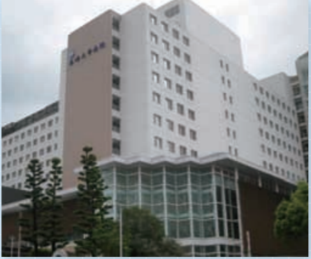
Nagasaki University Hospital, main building: Electrical fit-out (refurbishment)
