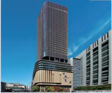
Nakanoshima Festival Tower: Air-conditioning installation
