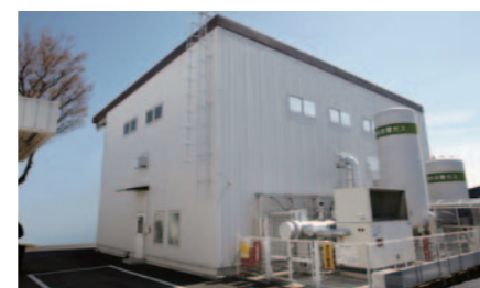
Second Experiment Building (Supercritical CO 2 plant)
