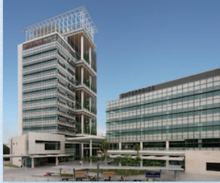
CREATE: Electrical fit-out, air-conditioning installation and plumbing
