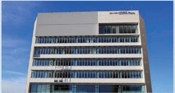
Public facility complex South Peer: Electrical fit-out
