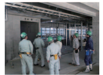
Inspection by the Health and Safety Cooperation Society
