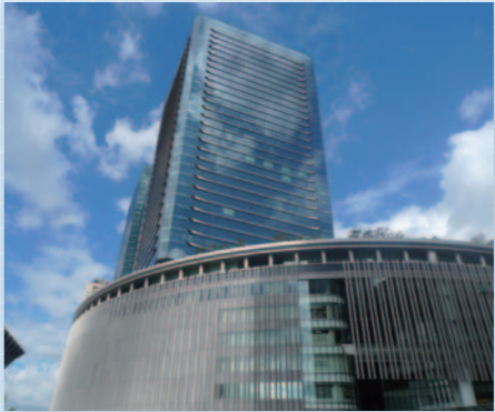
Grand Front Osaka South Building: Air-conditioning installation
