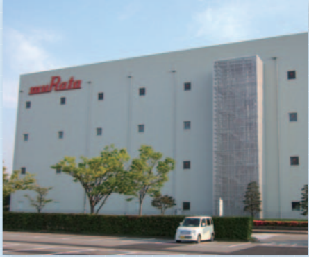
Toyama Murata Manufacturing, buildings C1 and C2: Air-conditioning installation (refurbishment)
