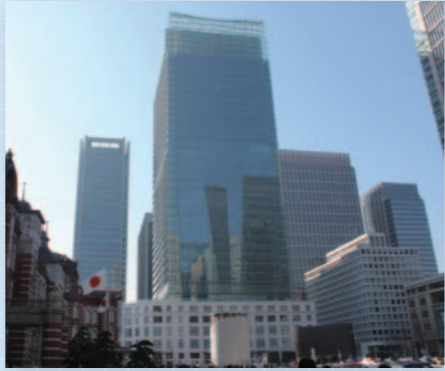
JP Tower: Air-conditioning installation
