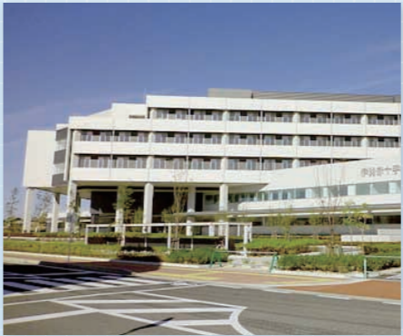
Japanese Red Cross Ise Hospital: Air-conditioning installation
