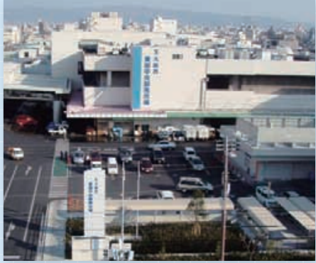
East Osaka Municipal Central Wholesale Market: Air-conditioning installation and plumbing
