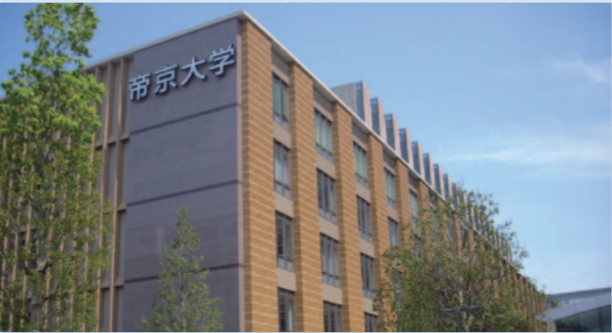
Teikyo University, Itabashi Campus building: Air-conditioning installation
