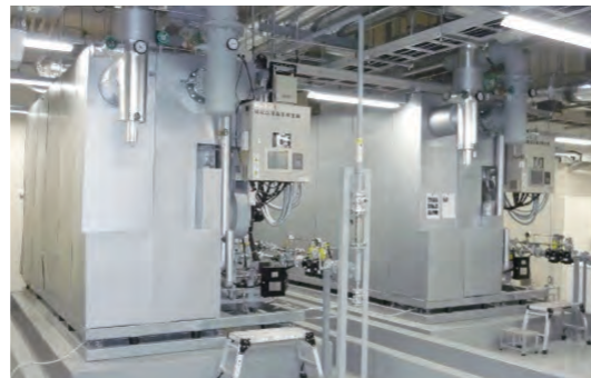
Gas-fired absorption-type cold/hot water supplier
