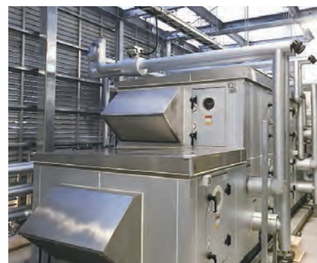
Desiccant air conditioner
