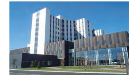
Obihiro Kosei Hospital (plumbing installation)
