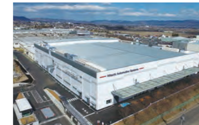
R&D Bldg. and Factory No. 5, Fukushima Plant Hitachi Automotive Systems (air conditioning and plumbing installations)
