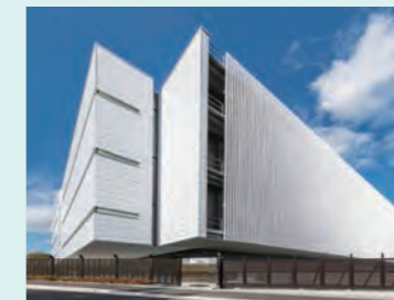
Installation example ② netXDC Sanda Center No. 2
