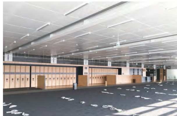
Indoor space with ceiling cooling panels
