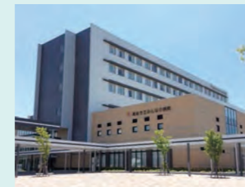
Installation example ① Takamatsu Municipal Hospital
