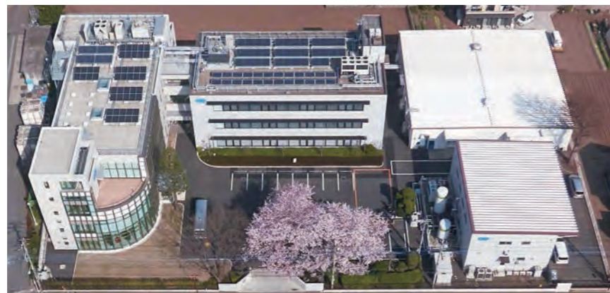
Aerial view of our Technical Research Laboratory in Miyoshimachi, Iruma-gun, Saitama Prefecture
