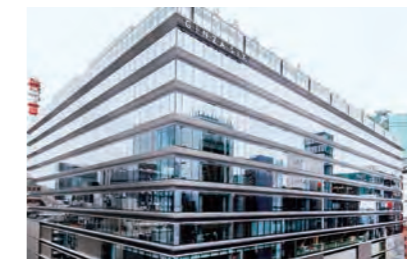
GINZA SIX (electrical installation)
