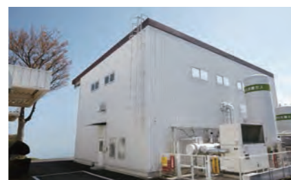
Supercritical CO 2 cleaning plant
