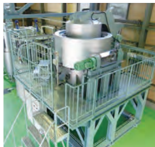
Supercritical CO 2 cleaning plant
