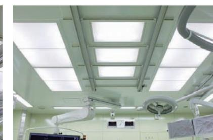
HEPA filter unit with built-in dimmable LED lighting
