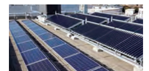
Solar heat collectors and solar panels
