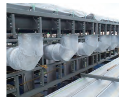
Through ducts and pipes installed in outer wall early into construction
