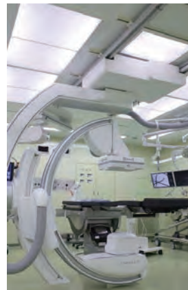
Hybrid operating room with HEPA filter unit featuring built-in dimmable LED lamp
