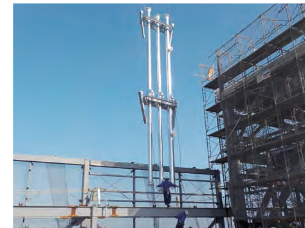
Riser unit in place
