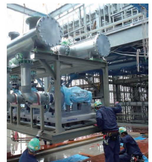
Pump unit for air conditioning machine room
