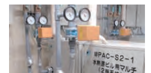
Water-source packaged air conditioning
