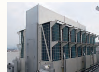
Air-cooled chiller silencer in service
