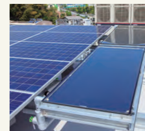
Photovoltaic panels/Solar heat collectors
