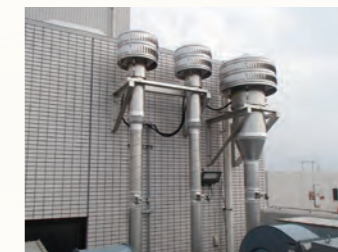
Ventilator fans for chemical exhaust system
