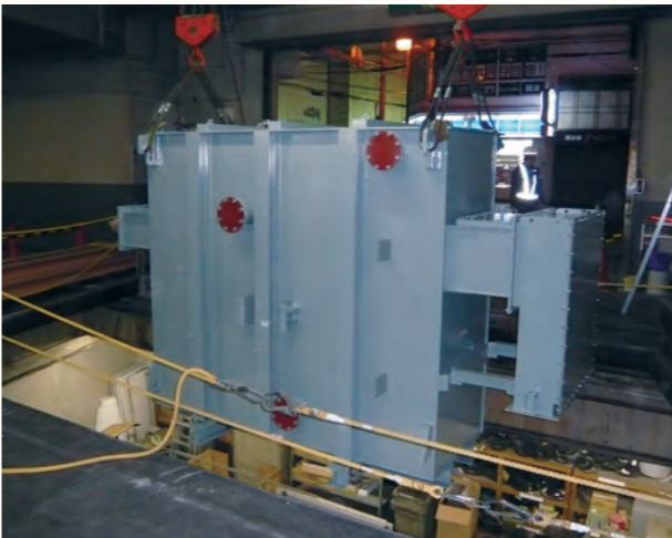
Carry-in of No. 3 extra-high-voltage transformer
