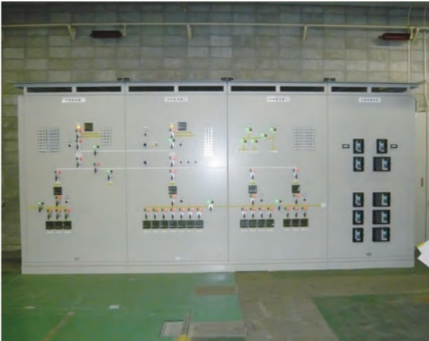
Extra-high-voltage monitoring panel
