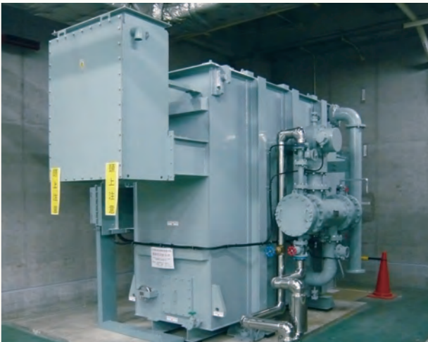
No. 3 extra-high-voltage transformer after installation
