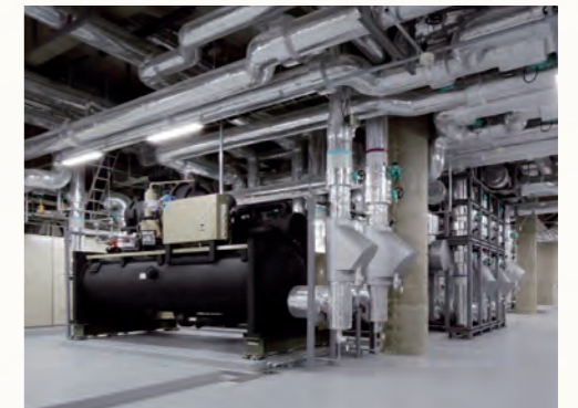
Heat source machine room (inverter turbo chiller)
