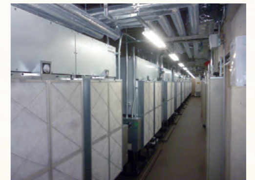
Air conditioning machine room (floor vent air handling unit)
