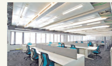
Radiant panels and lighting
