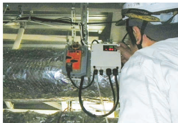
A room pressure control damper
