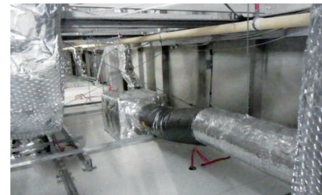
Maintenance access route above the ceiling clean panels
