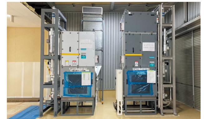
Air-conditioner-integrated piping unit
