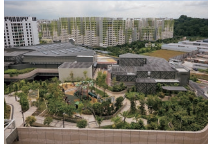
Housing and Development Tengah Park Centralised Cooling System (シンガポール)
